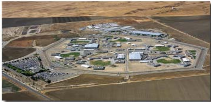
Aerial view of Avenal State Prison. Photo: CDCR
