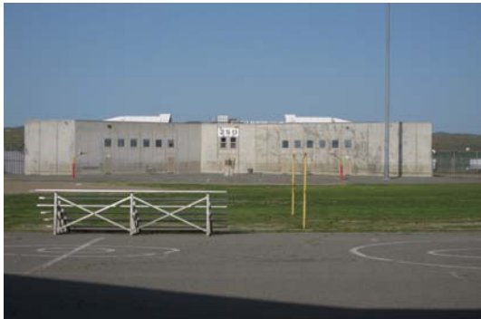
Figure 1 - Exterior View of Dorm Style Housing Unit. Photo: OIG, March 2010
